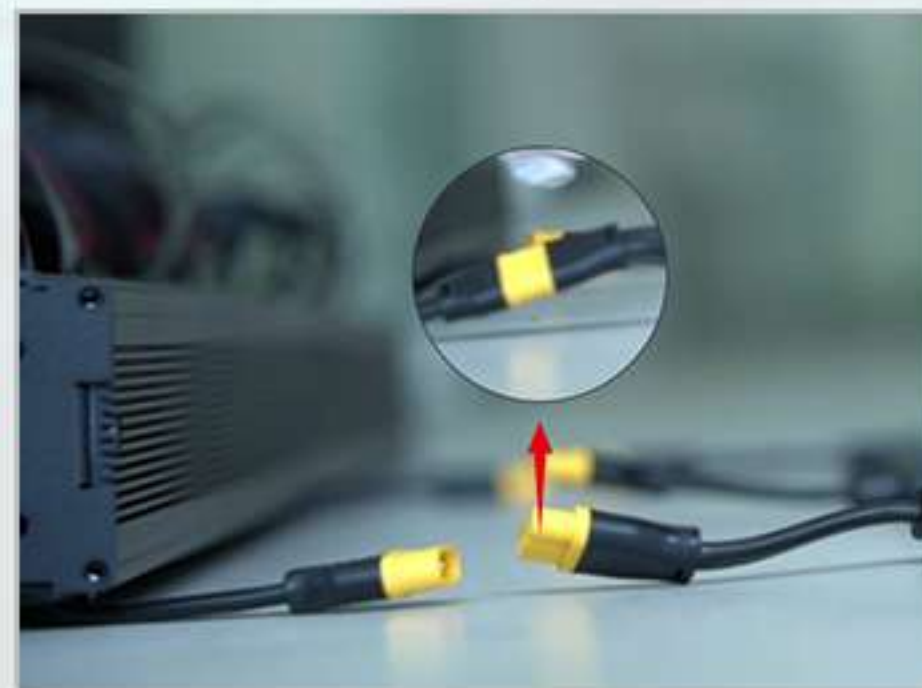
Step 6.End of installation of signal cables and power cables of the modules.
